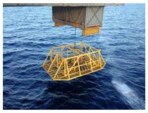
added: "The six steel DCTs, each weighing over 100 tonnes, complete with super-duplex piping manifolds, will enable the drilling of production and water injection wells without the need for rig moves for each cluster of wells. Delivery of the six structures is scheduled to take place during 2015 and Q1 2016 when they will then be installed on the seabed ready for use during Premier's drilling programme."
